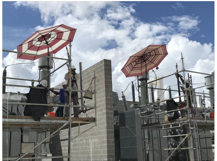
Battling the hot summer Texas sun while assembling terminations.
