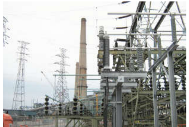
Completed G&W terminations.
