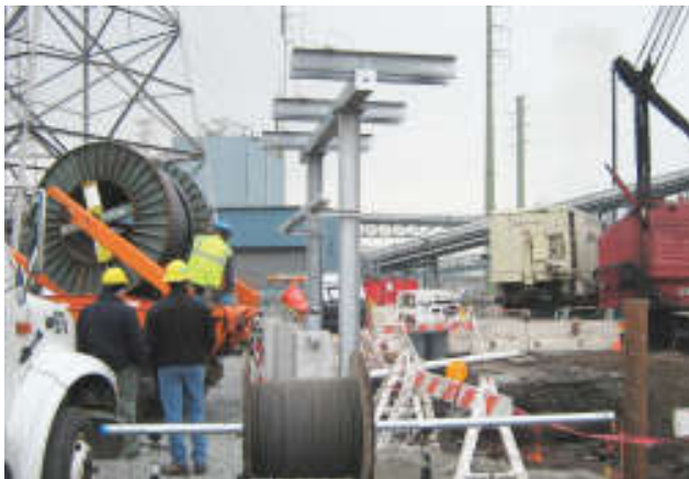
Pulling 138 kV cable.
