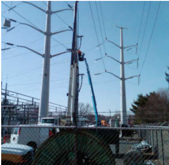
Demonstrated ability to safely install termination and cable near energized lines
