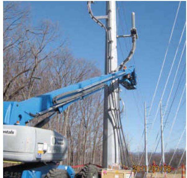
Completed terminations on 90ft pole
