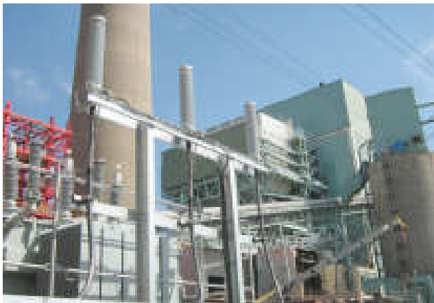
Completed HV terminations.
