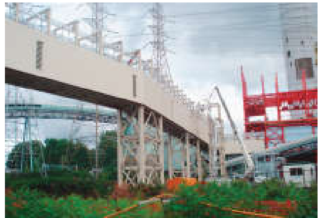
Cable pulled through tray.
