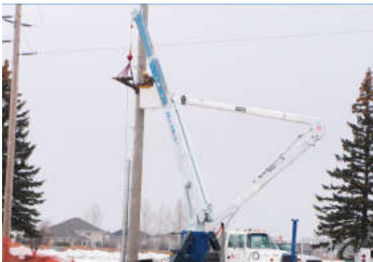
KCS technicians working on a 65 foot wooden pole from lift.
