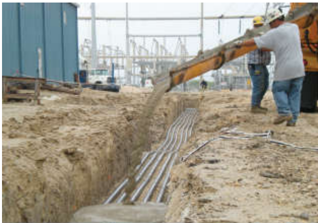
Installation of thermal backfill over direct buried cable.
