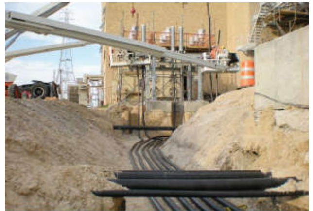
Direct buried under existing crossovers.
