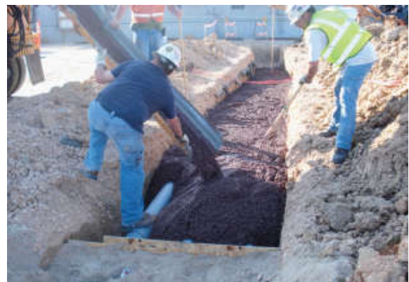
Installation of concrete encased duct bank.
