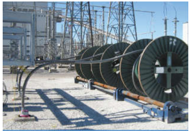
Cable pulled into ducts.
