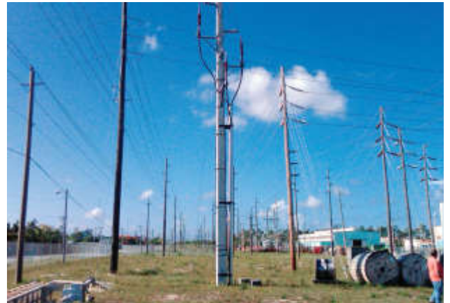
Pole with completed terminations.
