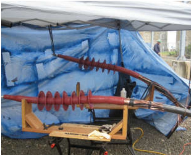
Completed high voltage termination.
