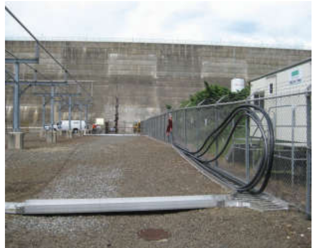
Cables with completed terminations temporarily fixed to the fence.
