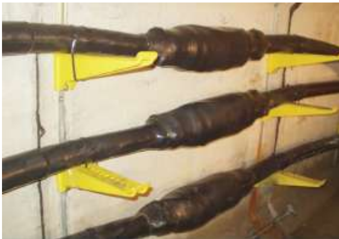
Completed 115 kV splices.
