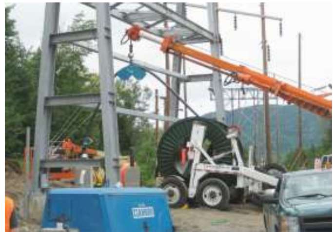
Pulling 115 kV cable.
