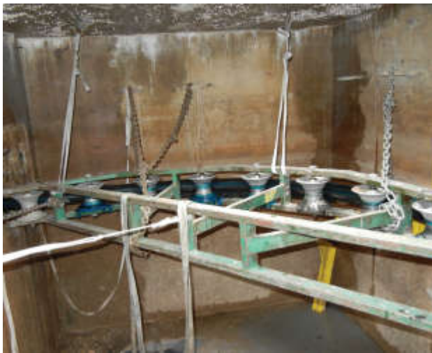
Pulling cable around corner in vault.
