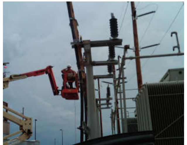
Jacket testing cable prior to cable prep.
