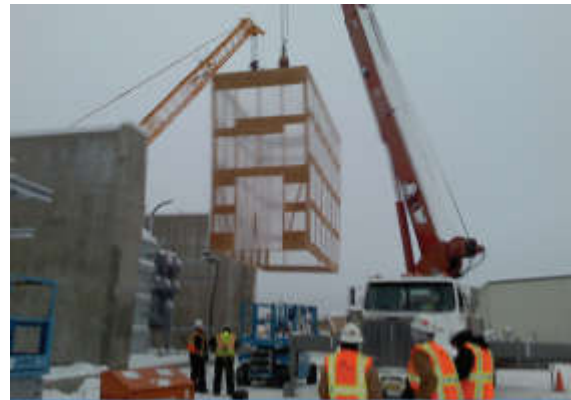
Setting of temporary shelter constructed on site in November and December
