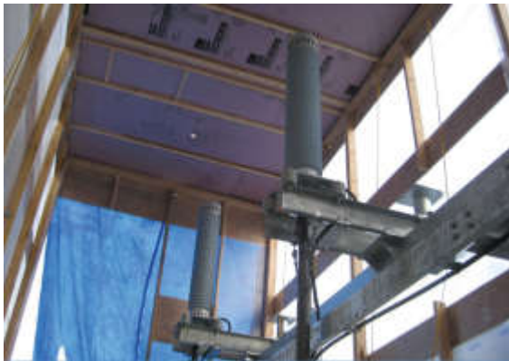
Completed terminations inside of temporary shelter
