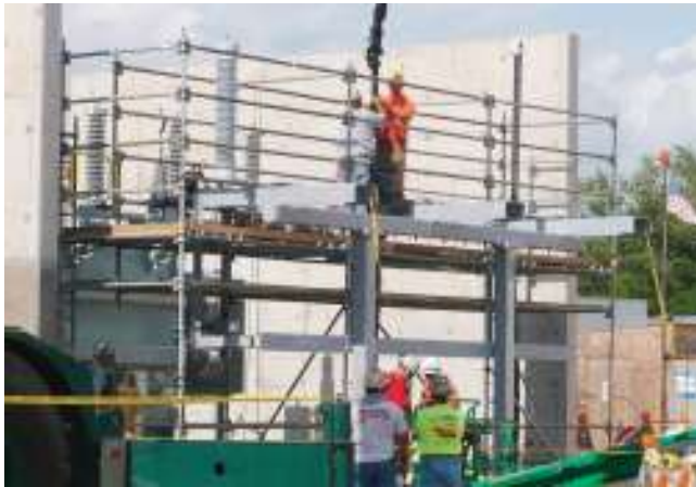
KCS technicians building HV terminations.
