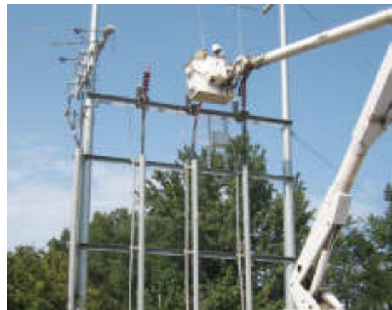
Completed 69kV heat shrink termination.
