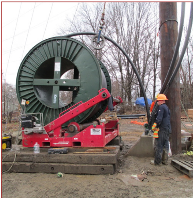
115kV 2000 kcmil cable being pulled into existing ducts.
