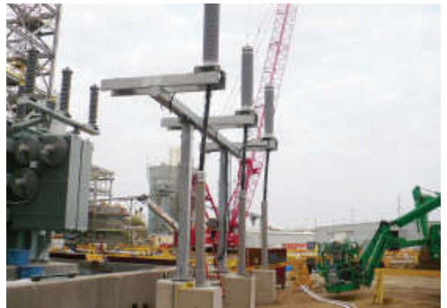
Completed HV terminations.
