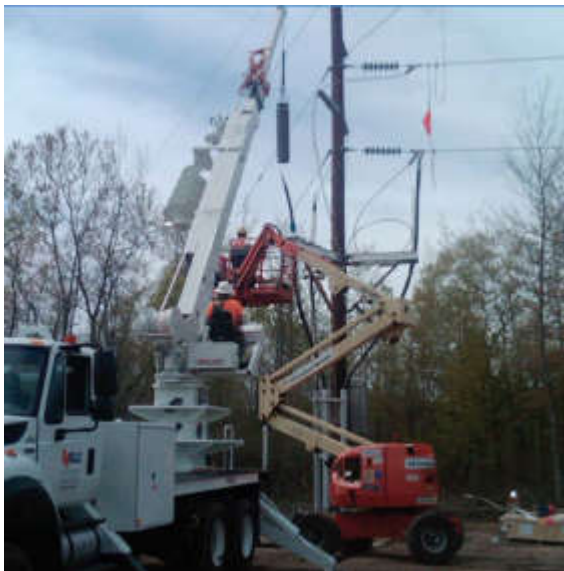
Setting of high voltage termination
