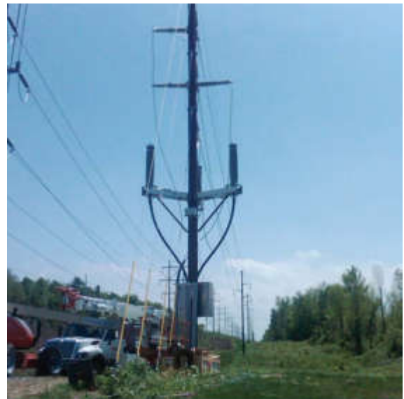
Completed high voltage termination
