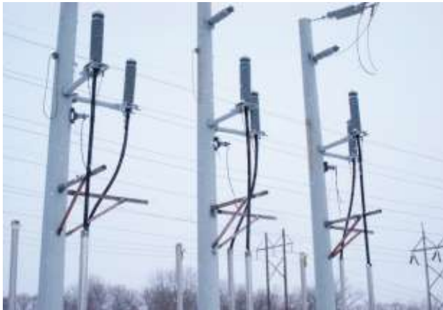
Completed HV termination.
