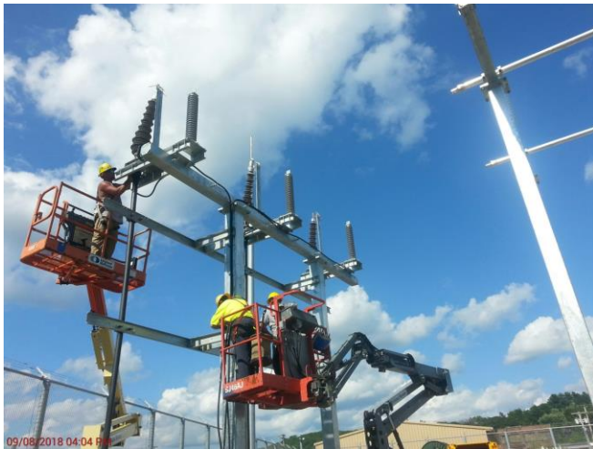
Assembling G&W Dry Type Terminations
