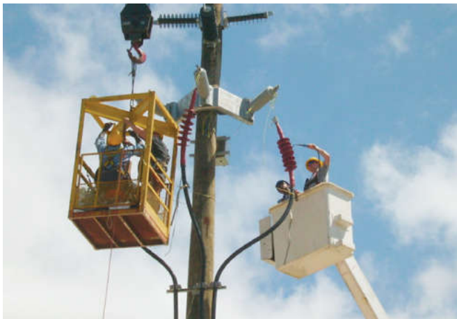
Termination Installation
