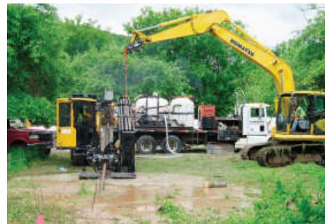
28 Inch diameter directional bore.
