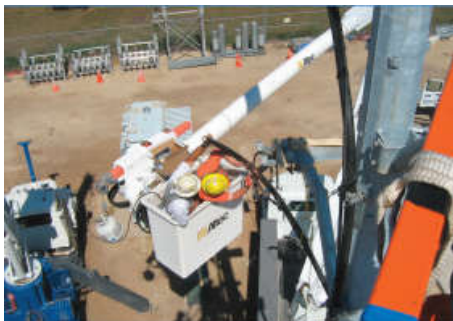
KCS technician making 69 kV termination.
