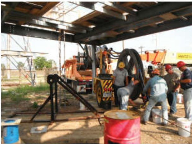
Pulling three cables into a single 6 inch conduit.
