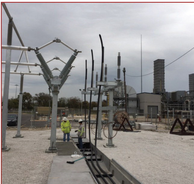
Laying cable in concrete trench
