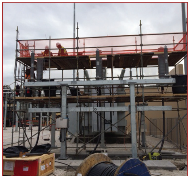
Technicians working to assemble G&W PAT 140 terminations on scaffolding
