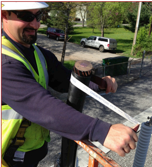
Prepping the cable for 10kV jacket test.
