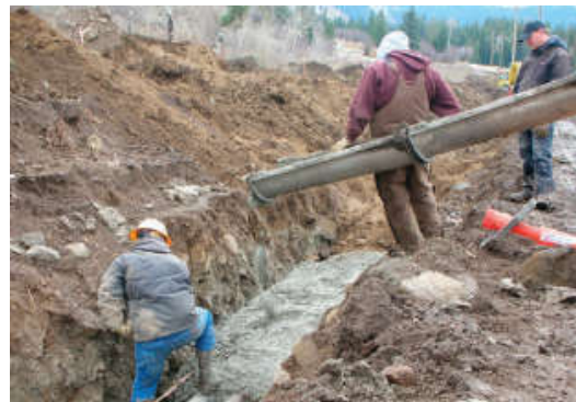
Ductbank Construction
