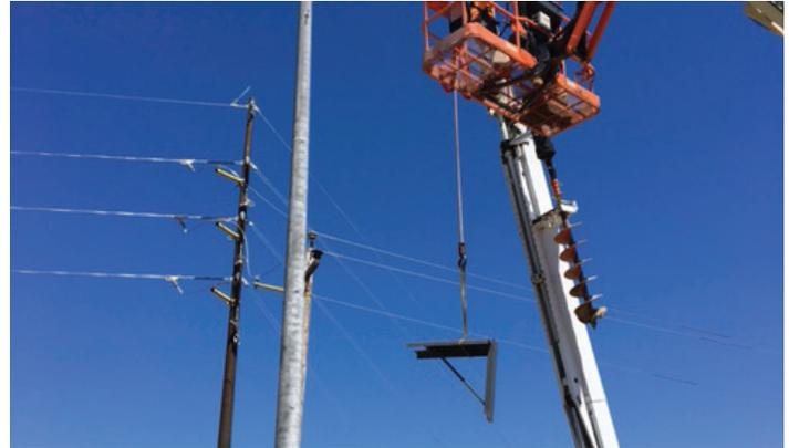
Termination brackets being installed on one of the two pre-cast riser poles.
