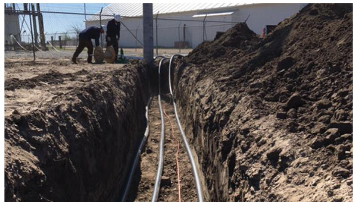
The 600 foot trench housed the 3 phases of the 69kV cable.
